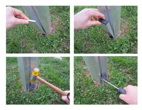
b) Set mounted goal with fixed ground sockets in the foundations (80x80x100cm). To enable a drain off of possible water we recommend to stick a tube each below the boreholes of the ground sockets.
