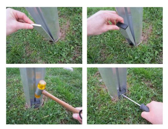
b) Set mounted goal with fixed ground sockets in the foundations (80x80x100cm). To enable a drain off of possible water we recommend to stick a tube each below the boreholes of the ground sockets. After careful adjustment of the goal to the side and specified height by crossed bars pour concrete into the foundation ditches.
