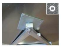
Stick 1 washer  $\emptyset$  outside 28mm, DIN 125-1 on the provided screwing device and screw it firmly into the thread of the plug plate. Make sure that the reel can move freely.
